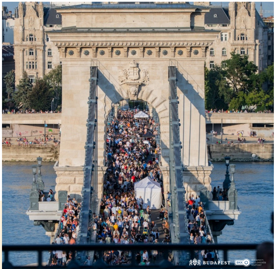
Pedestrian crossing the newly refurbished Chain Bridge
