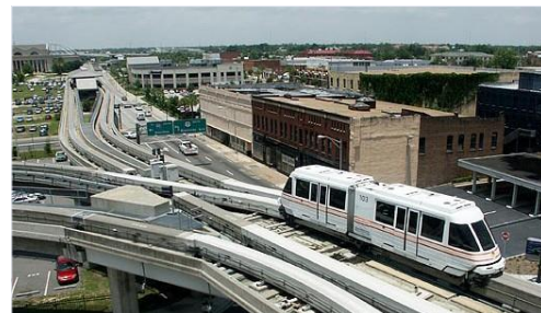
Figure 10.5. Monorail System. Photo courtesy of Flickr/Jon Bell
