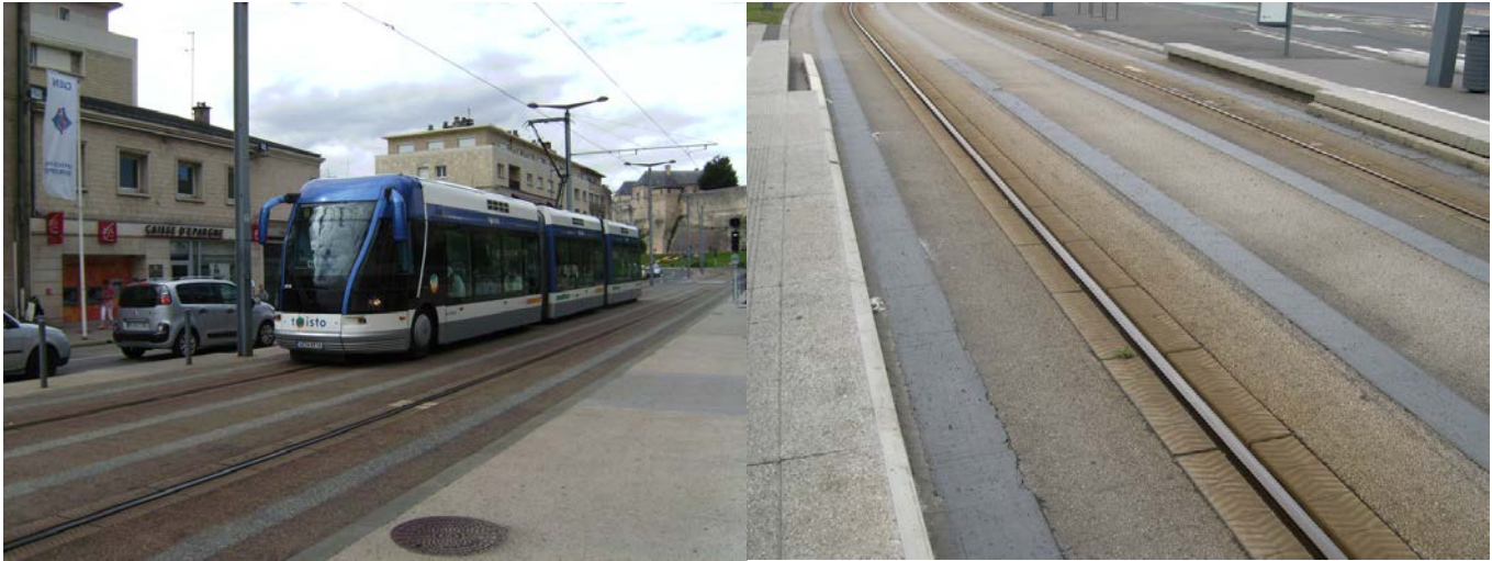
Left: Rubber-tyre tramway in Caen, France. Right: Guiderail for a conventional rubber tyred tramway.
